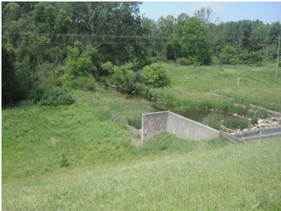
Plate 22: Topography, Morrison Dam Below Morrison Lake and Steep Slope, From Morrison Line, Facing Northwest
