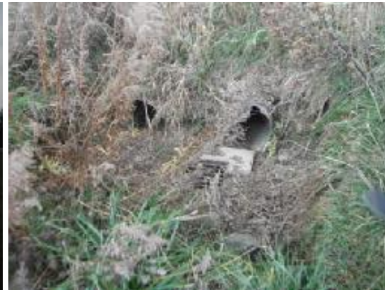
Photograph 2. Tile drain Goshen Line ↑
