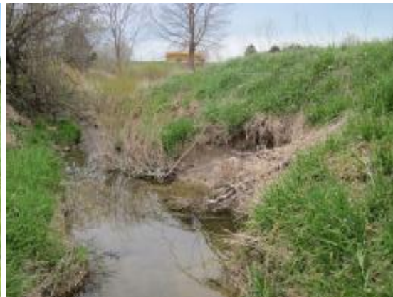
Photograph 2. Site overview east ↑
