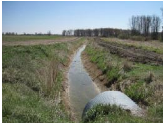
Photograph 1. Site overview south ↑
