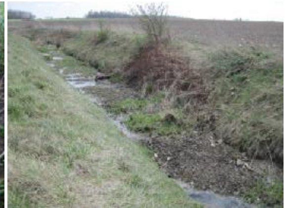
Photograph 3. Low flow barrier ↑
