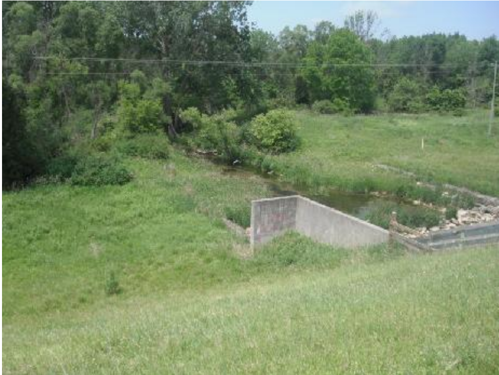
Plate 12: Morrison Dam, east of Exeter, looking downstream from Morrison Line.
