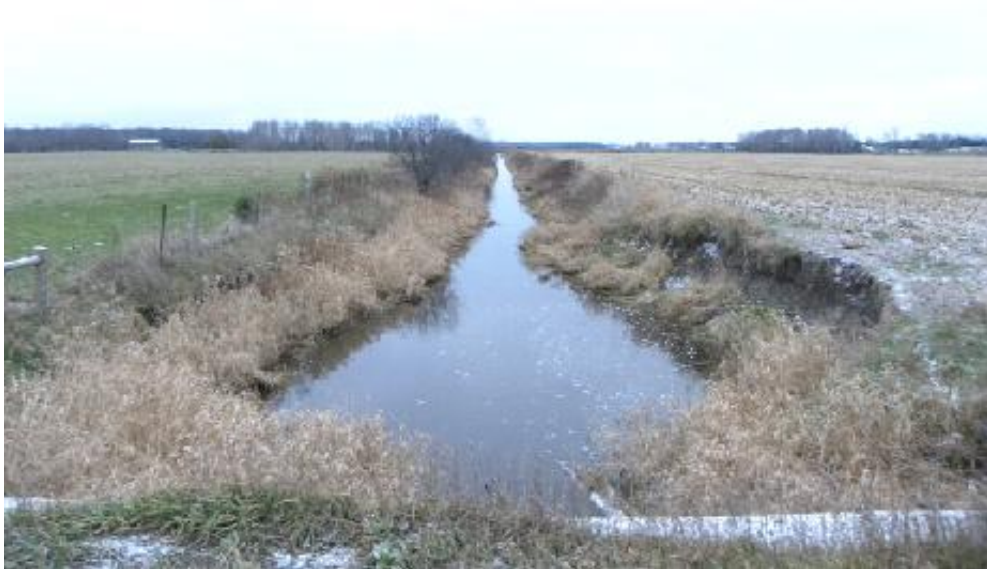
Plate 9: Drainage ditch crossing beneath the Zurich Hensall Road between Parr Line and Babylon Line, looking south.
