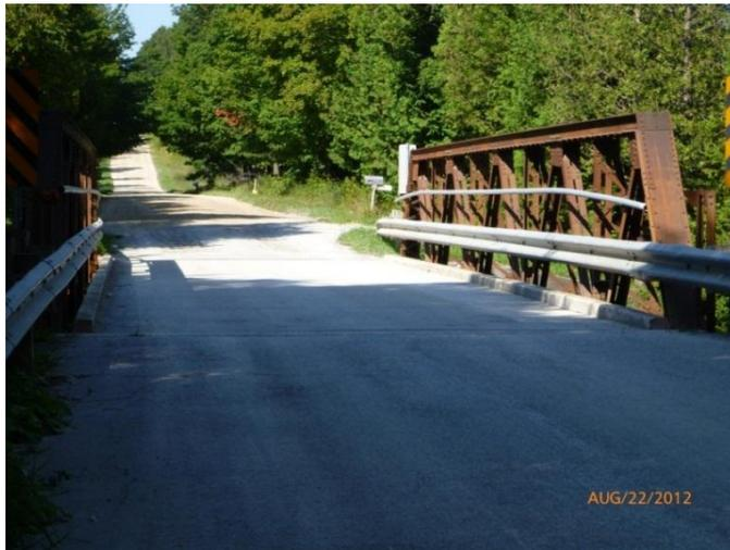
**Description** - This is a Warren pony truss bridge, with the typical configuration of the diagonal members of the truss repeating themselves as a series of “Ws”. There is a reinforced steel guard rail on the interior (roadside) of both sides of the bridge. The 2 lane gravel roadway narrows to 1½ lanes at the bridge.
