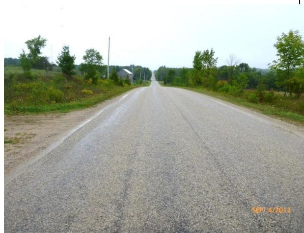
**Description** - chip stone and tar, 2 lane roadway, narrow gravel shoulders and shallow ditches, gently rolling hill topography.
