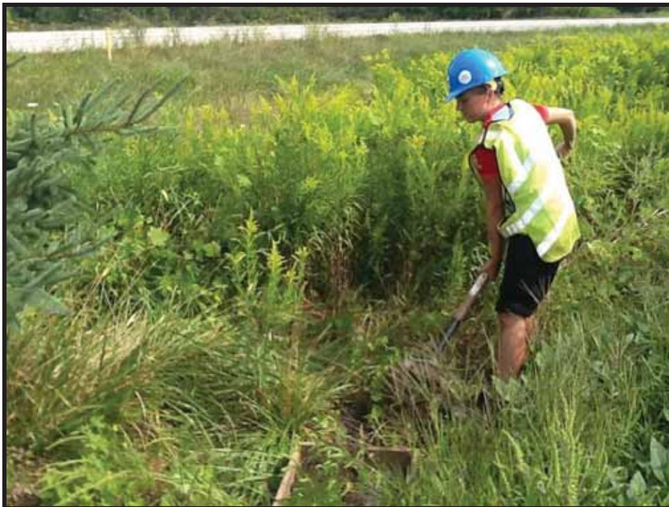
**Image 128: View of Crewmember Test Pitting at a Maximum 5 m Interval at GSH1605 (East)**
