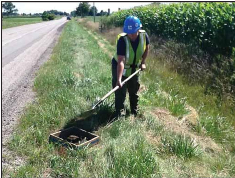
**Image 106: View of Crewmember Test Pitting to Confirm Disturbance at GSH1498/1659**
