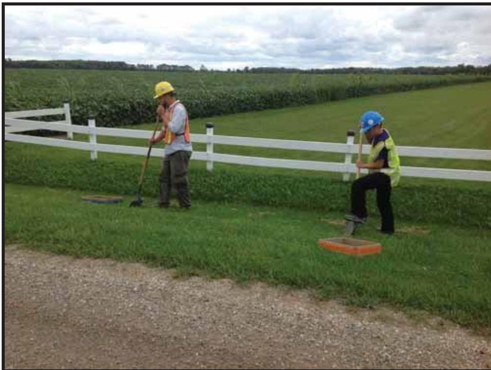
**Image 82: View of Crewmembers Test Pitting to Confirm Disturbance at GSH1095**
