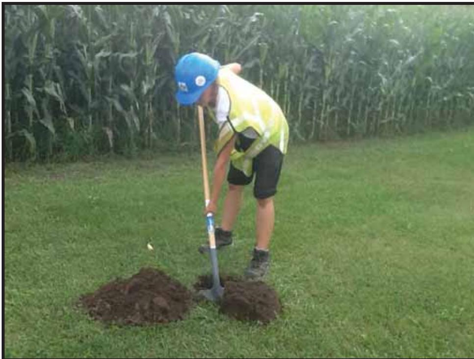
**Image 76: View of Crewmember Test Pitting to Confirm Disturbance at GSH1077**
