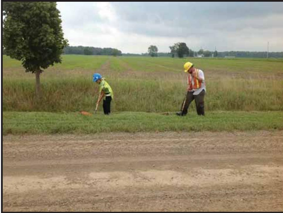
**Image 13: View of Crewmember Test Pitting to Confirm Disturbance at GSH1020**
