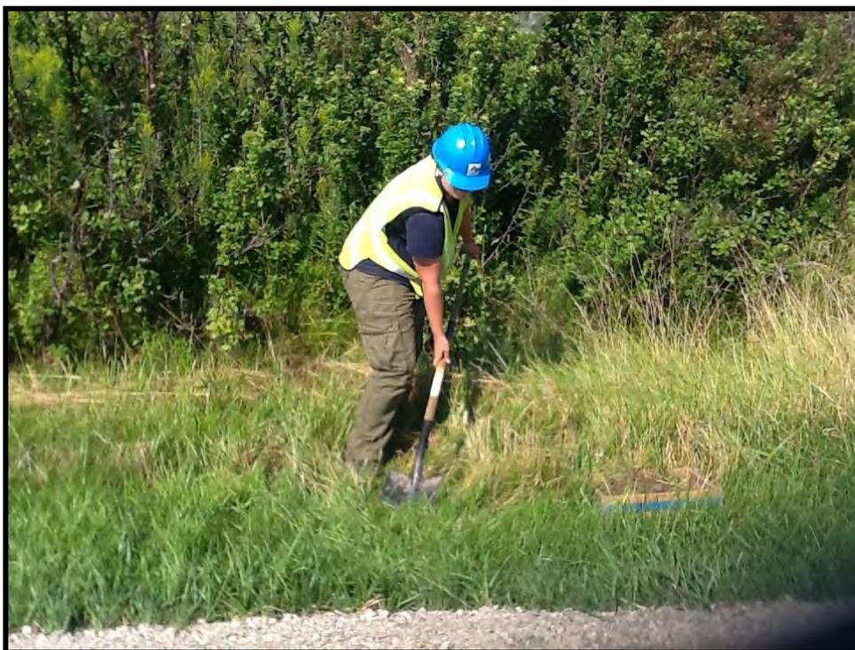
**Image 144: View of Crewmember Test Pitting to Confirm Disturbance at GSH1758**
