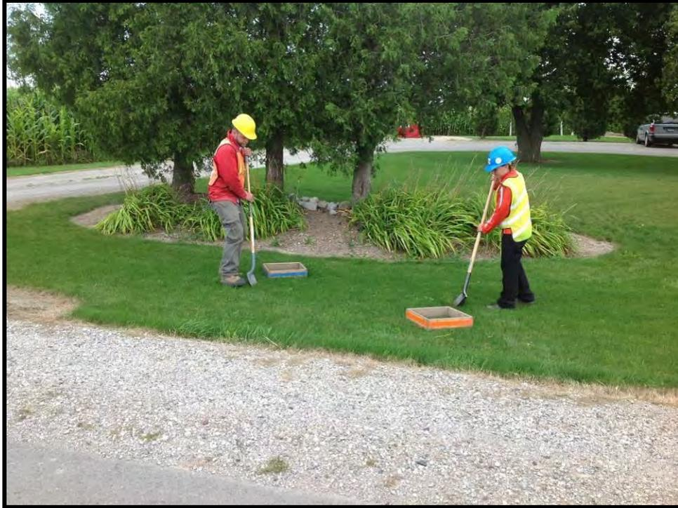
**Image 163: View of Crewmembers Test Pitting to Confirm Disturbance at GSH2056
