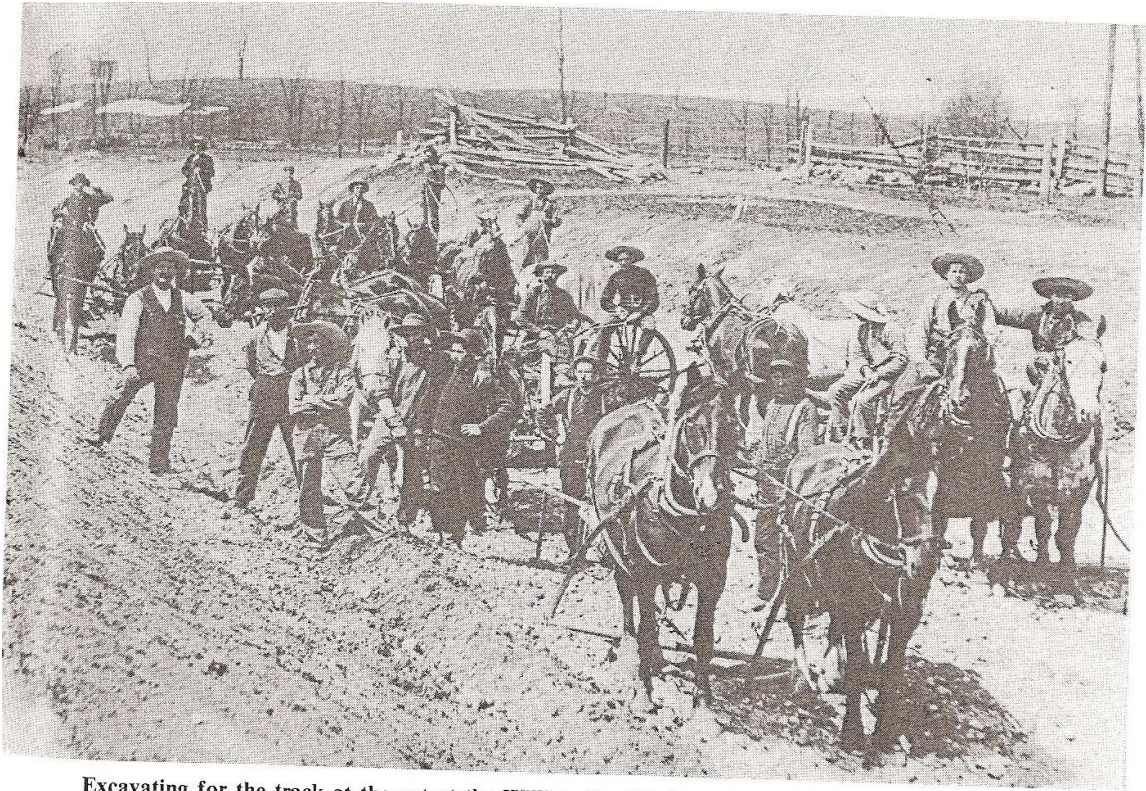
Excavating for the track at the cut at the William Smellie farm, Lot 31, Concession 1, N.D.R.
