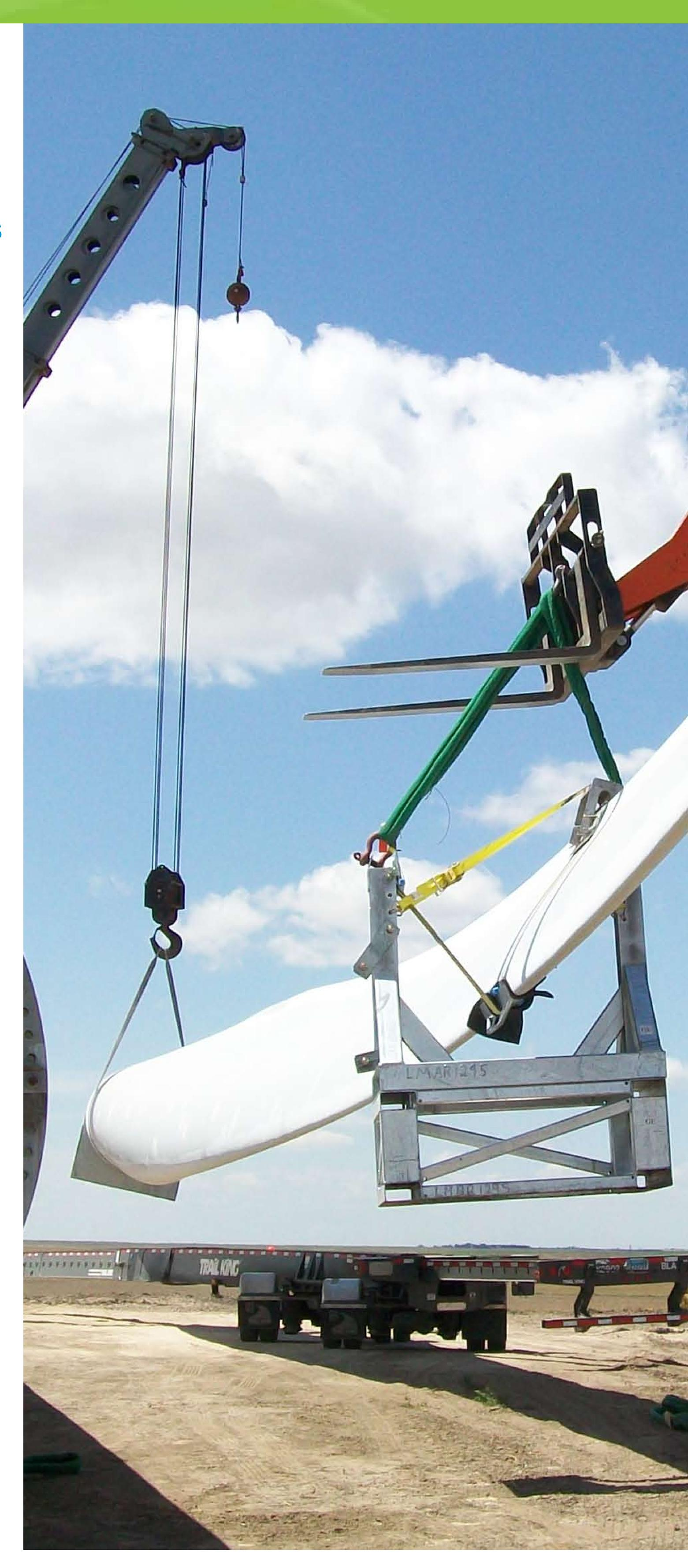
• Repair, refurbishment and replacement of turbines is typical of a preventative maintenance program
