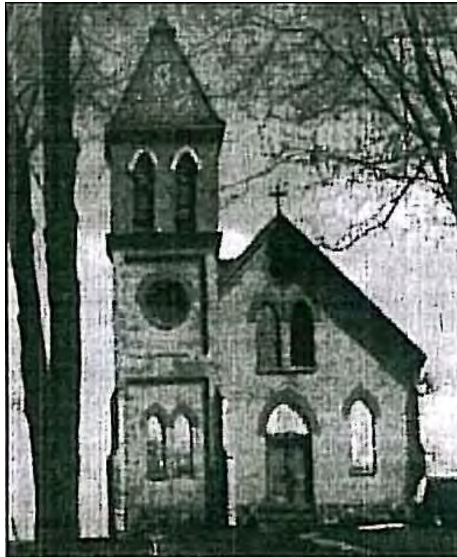
Plate 7: St. Patrick's Church, Adelaide Village, date unknown, demolished in 1984 (ATHG 2001: 460).
