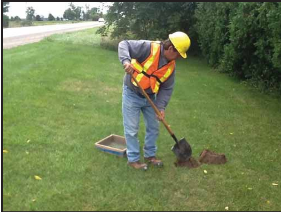
Image 201: View of Crewmember Test Pitting to Confirm Disturbance at Grand Bend Line from GSH1528 to GSH1016 (North) (Photo Taken September 3, 2013; Facing South)
