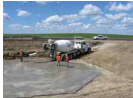
A cement truck delivers cement to a foundation.
