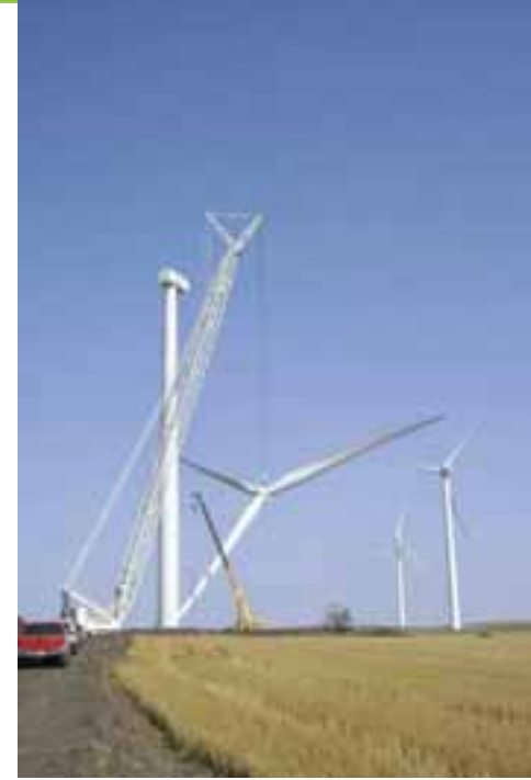
Cranes lift a rotor to be installed on the nacelle at the top of the tower.
