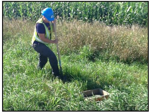
Image 168: View of Crewmember Test Pitting to Confirm Disturbance at GSH2108 (Photo Taken August 9, 2013; Facing South)
