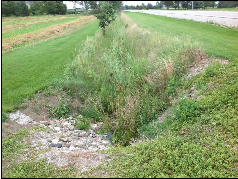
Image 121: Area of No Archaeological Potential – Disturbed Lands at GSH1526 (Photo Taken August 13, 2013; Facing South)
