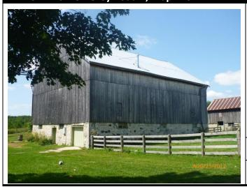
**Description** — There is a single car garage, frame construction with a rooster weather vane; a small barn with a metal roof and wooden addition. The small barn has a concrete foundation and vertical wooden barn board. The house sits on a fieldstone foundation.
