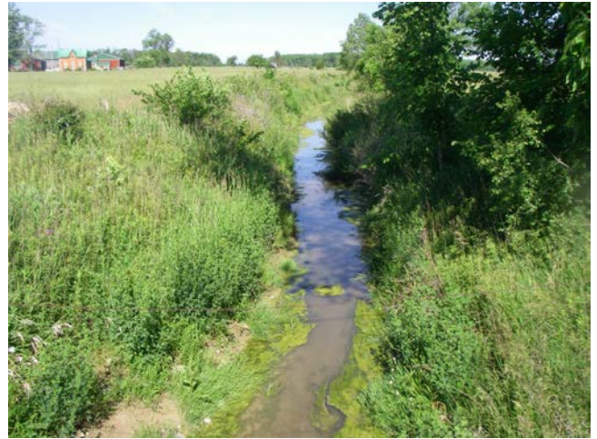
Photo 8 Station 14-2 – Woods Creek (Spring 2012) – Facing downstream (west) showing a channel overview.
