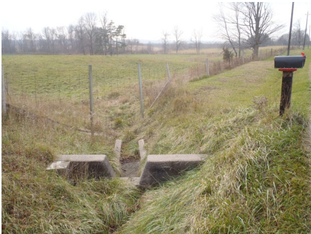
Photo 17 Station 31-4 – Cates Drain (Fall 2011) - Facing downstream (southwest) showing dry culvert for conveying roadside and surficial drainage.
