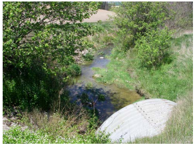
Photo 16 Station 24-1 – Bannister Drain (Spring 2012) – Facing downstream (northwest) showing channel overview.
