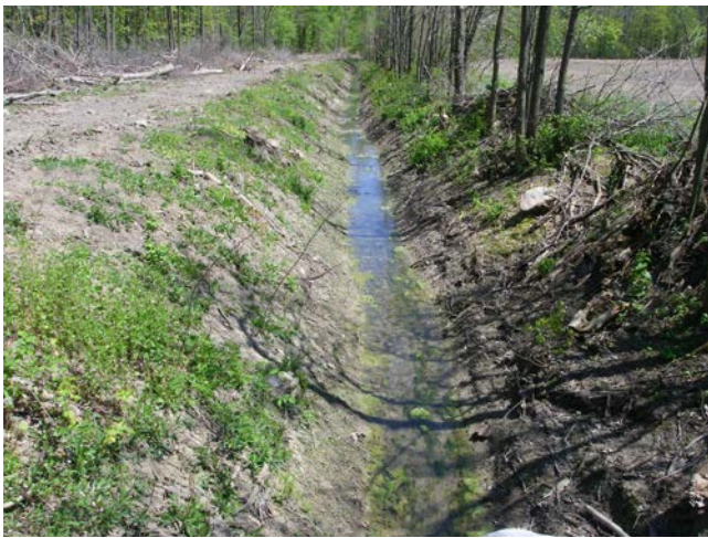
Photo 3 Station 23-1 – 30 Creek Drain (Spring 2012) – Facing upstream (southeast) showing recently cleared channel.
