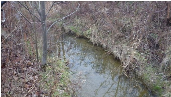
Photo 17 Station 22-6– Bannister Drain (Fall 2012) – Facing upstream from station showing channel overview.
