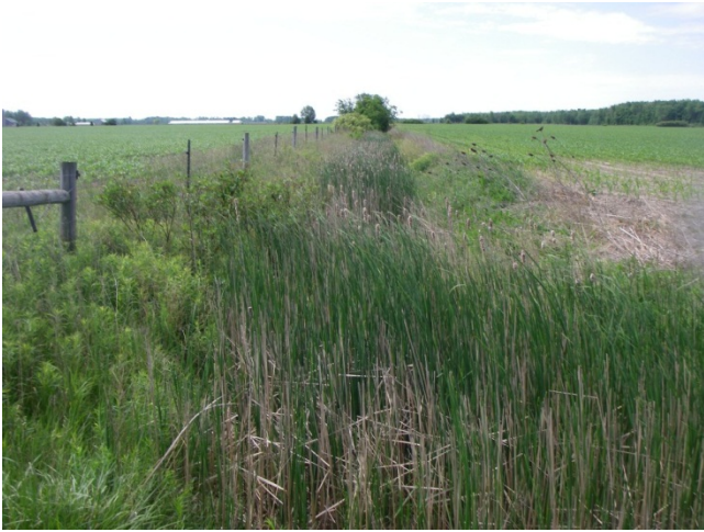
Photo 13 Station 1-3 – Walden Drain (Summer 2012) - Facing upstream (south) from Ravenswood Line showing channel and adjacent agricultural field.
