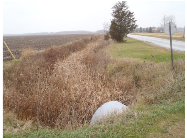
Photo 16 Station 31-1 – Hartley Drain (Fall 2011) - Facing downstream (north) along the west side of Hillsboro Road showing culvert and channel densely lined with cattails.
