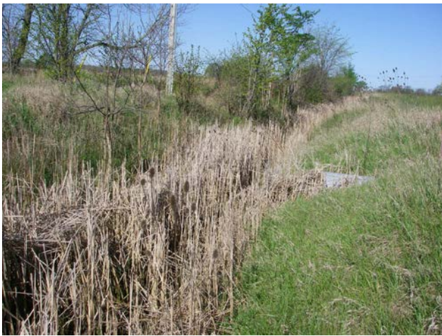
Photo 9 Station 25-2 – Greendees Drain (Spring 2012) – Facing downstream (west) showing cattail lined channel.
