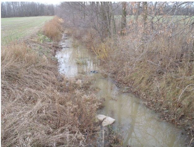
Photo 15 Station 4-1 – Ross Drain (Fall 2011) - Facing upstream (east) along Thomson Line showing culvert and channel overview.
