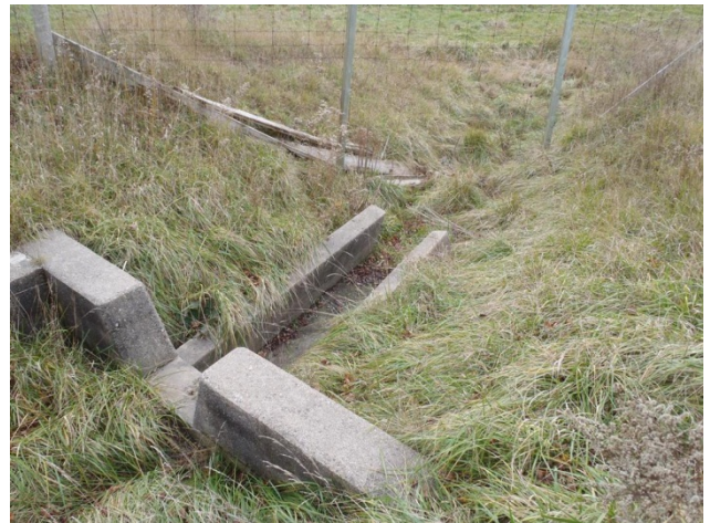
Photo 18 Station 31-4 – Cates Drain (Fall 2011) - Close-up of downstream culvert.
