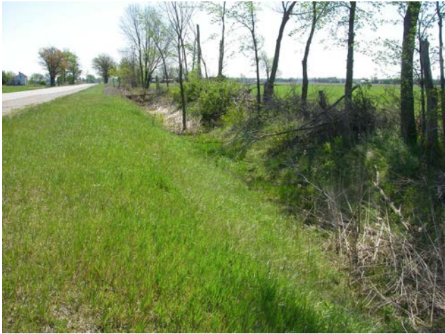
Photo 1 Station 16-5 – Anderson Drain (Spring 2012) – Facing upstream (southeast) along Townsend Line showing incised channel and cattails.
