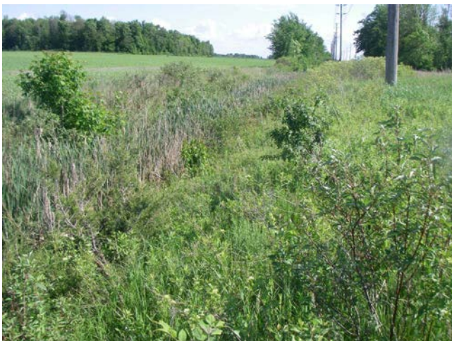
Photo 11 Station 52-1 – McCallum Drain (Spring 2012) – Facing upstream (south) along Elarton Road showing
