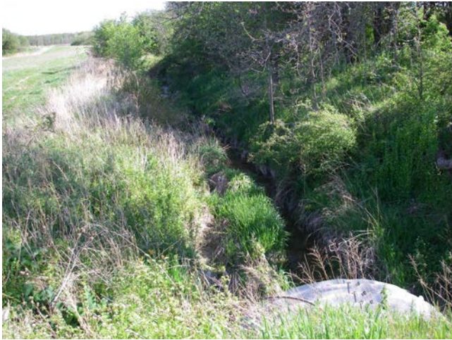
Photo 7 Station 31-2 – James-Wilkinson Drain (Spring 2012) – Facing upstream (south) showing channel and surrounding vegetation.
