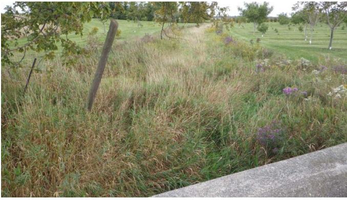
Photo 19 Station 60-1 – Kernohan-O'Donnell Drain (Fall 2012) – Facing upstream showing channel overview.
