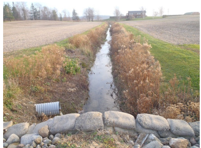
Photo 11 Station 19-1 – McKinley Drain (Fall 2011) - Facing upstream (south) from Hubbard Line showing culvert, tile drainage inputs and channel overview.
