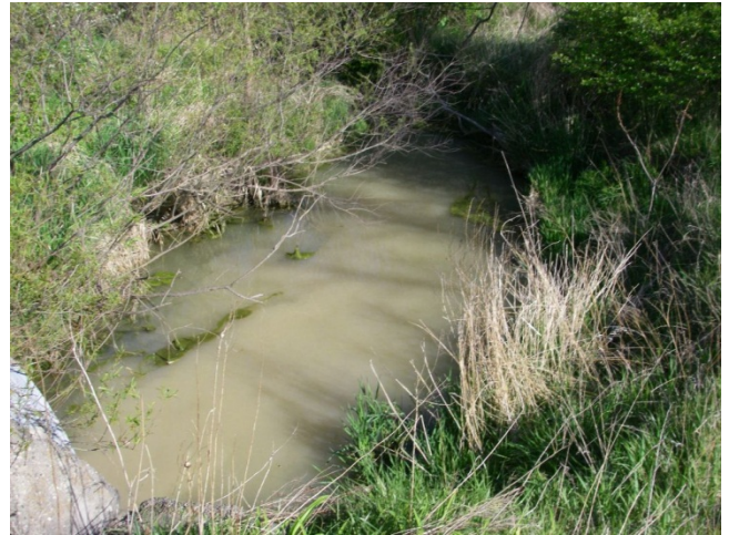
Photo 14 Station 19-1 – McKinley Drain (Spring 2012) – Facing downstream (north) showing channel and culvert.
