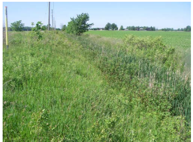
Photo 12 Station 52-1 – McCallum Drain (Spring 2012) – Facing downstream (north) along Elarton Road showing cattail lined channel.
