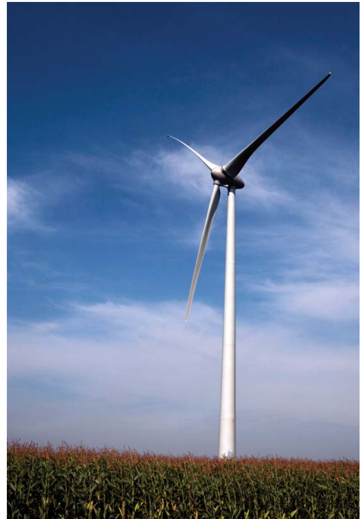
Enercon Turbine at Ripley
