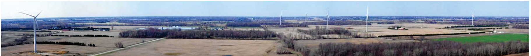
Kent Breeze Wind Power Project
