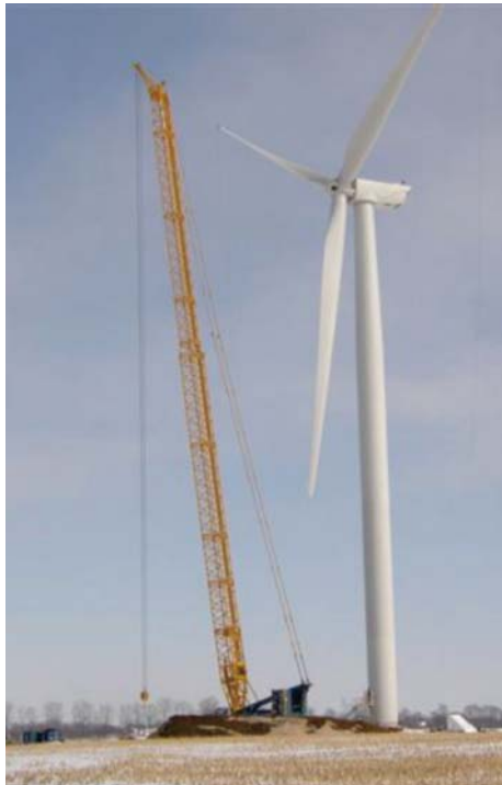
Recently erected wind turbine at Kent Breeze Wind Power Project
