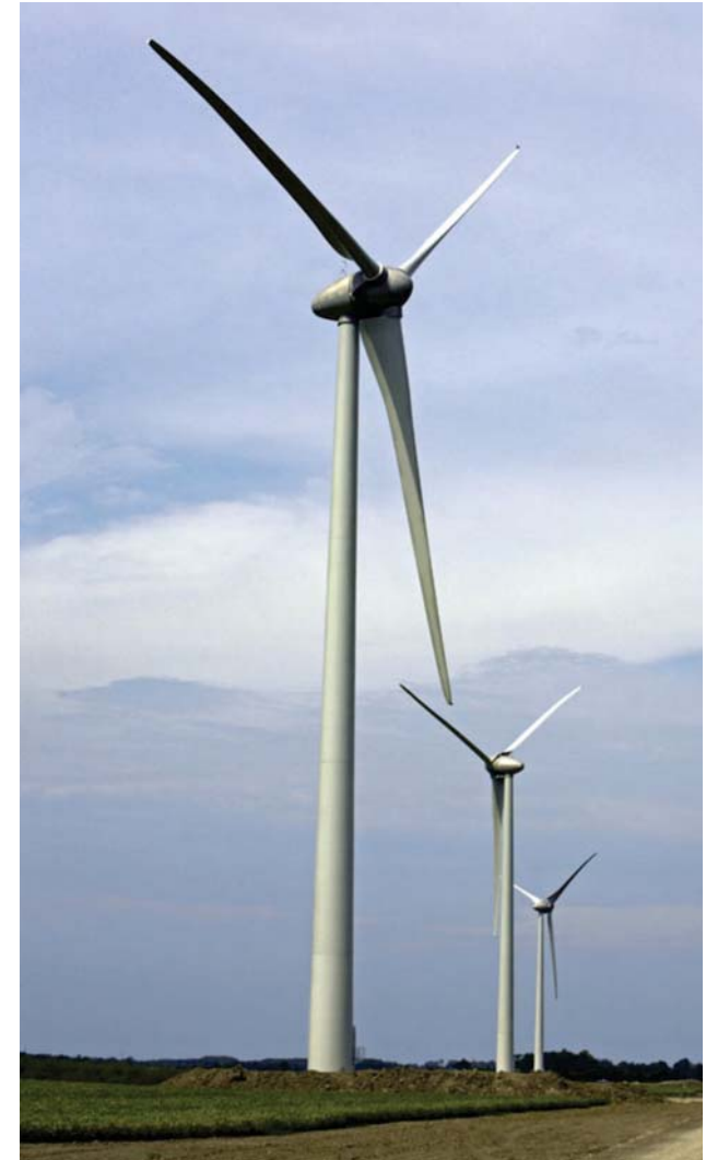
Recently erected wind turbines at Ripley Wind Power Project
