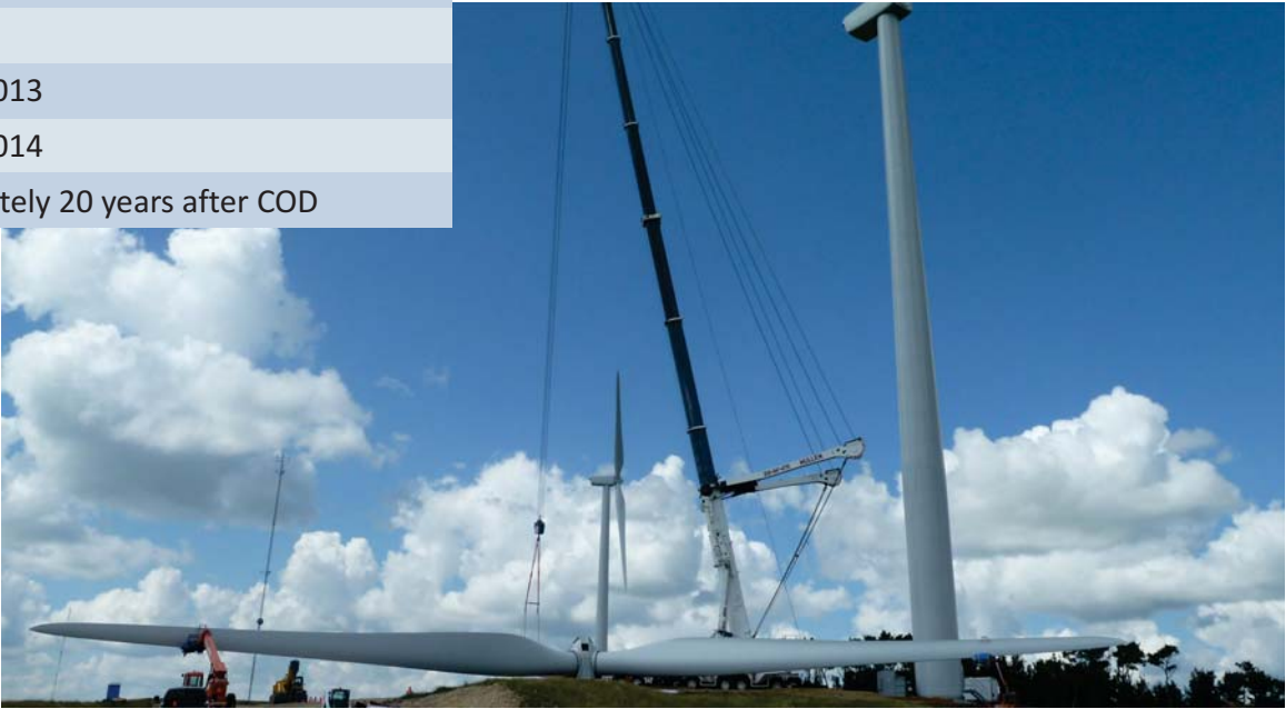
Preparation of rotor installation - Wintering Hills Wind Power Project
