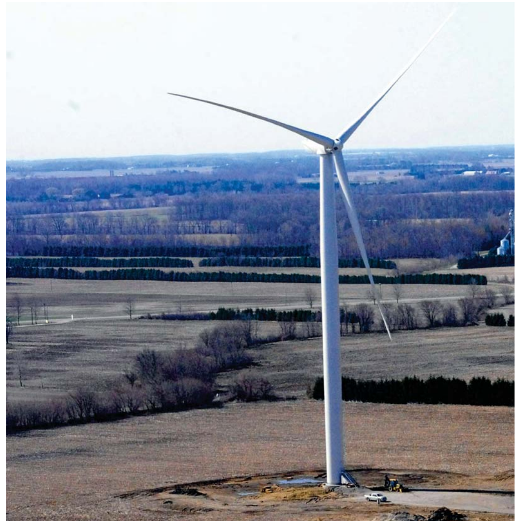
First GE 2.5 MW turbine in North America - Kent Breeze Wind Power Project
