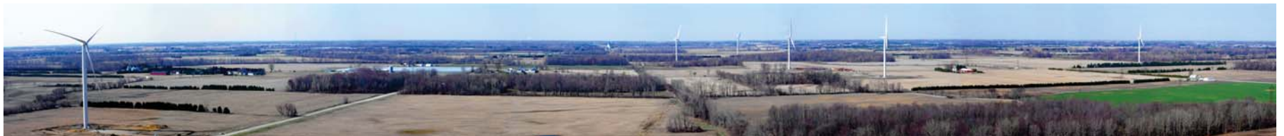
Kent Breeze Wind Power Project
