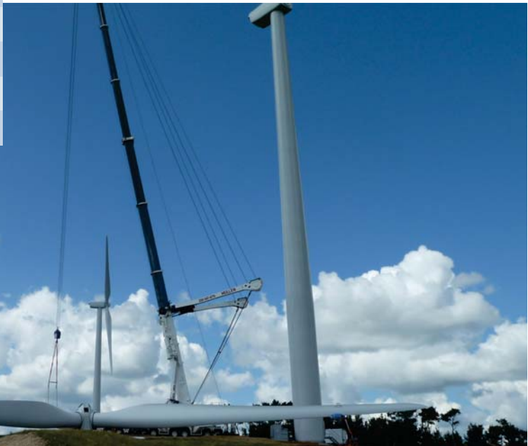
Preparation of rotor installation - Wintering Hills Wind Power Project
