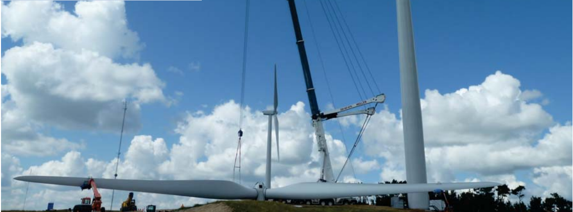
Preparation of rotor installation - Wintering Hills Wind Power Project
