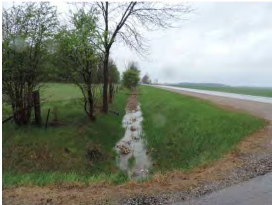
Photo 1 Southwest Corner of Townsend Line and Uttoxeter Road
