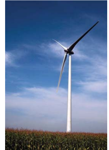
Enercon Turbine at Ripley
