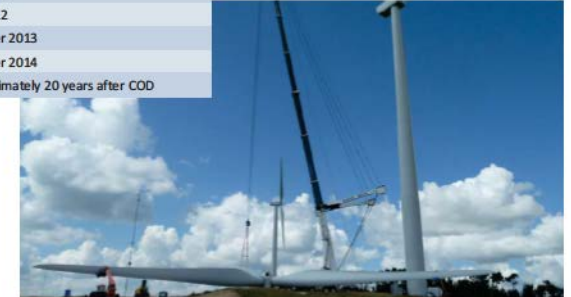
Preparation of tower installation - Whiting Hills Wind Power Project
