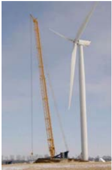
Recently erected wind turbine at Kent Breeze Wind Power Project
