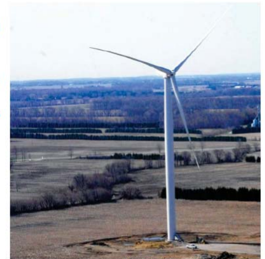
First GE 2.5 MW turbine in North America – North Brains Wind Power Project
