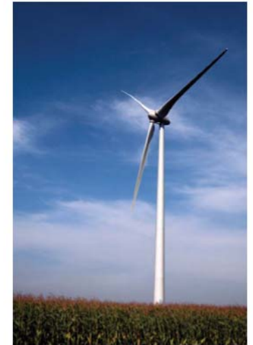
Enercon Turbine at Ripley
