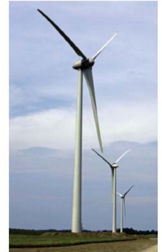
Recently erected wind turbines at Ripley Wind Power Project
