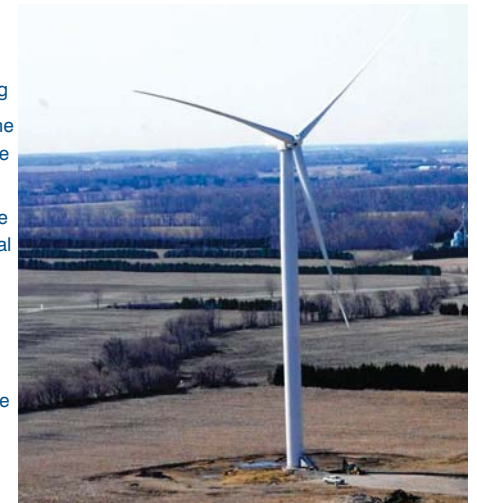
First GE 2.5 MW turbine in North America - Kent Breeze Wind Power Project
