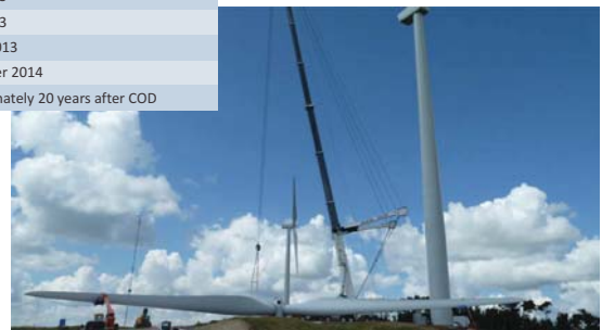
Preparation of rotor installation - Withering Hills Wind Power Project
