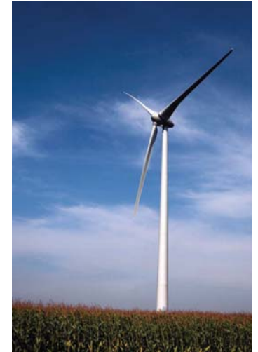
Enercon Turbine at Ripley
