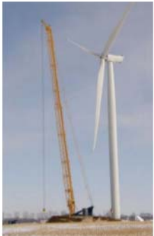
Recently erected wind turbine at North Brains Wind Power Project
