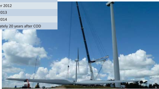
Preparation of rotor installation – Withering Hills Wind Power Project
