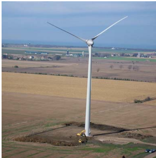
Ripley Wind Power Project
