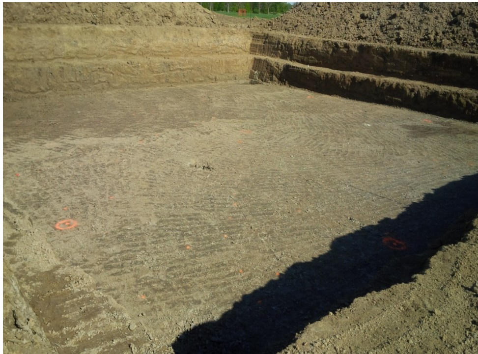
Photo 1 – CP210 – Foundation Subgrade
