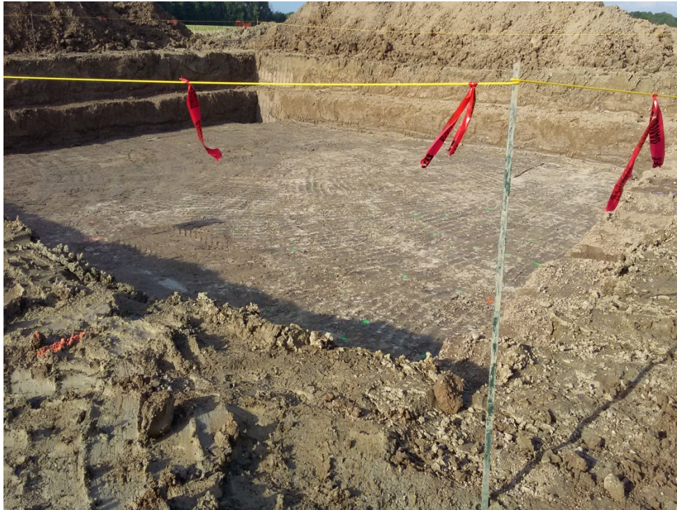
Photo 5 – CP245– Foundation Subgrade
