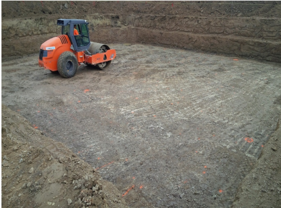
Photo 4 – CP244– Foundation Subgrade
