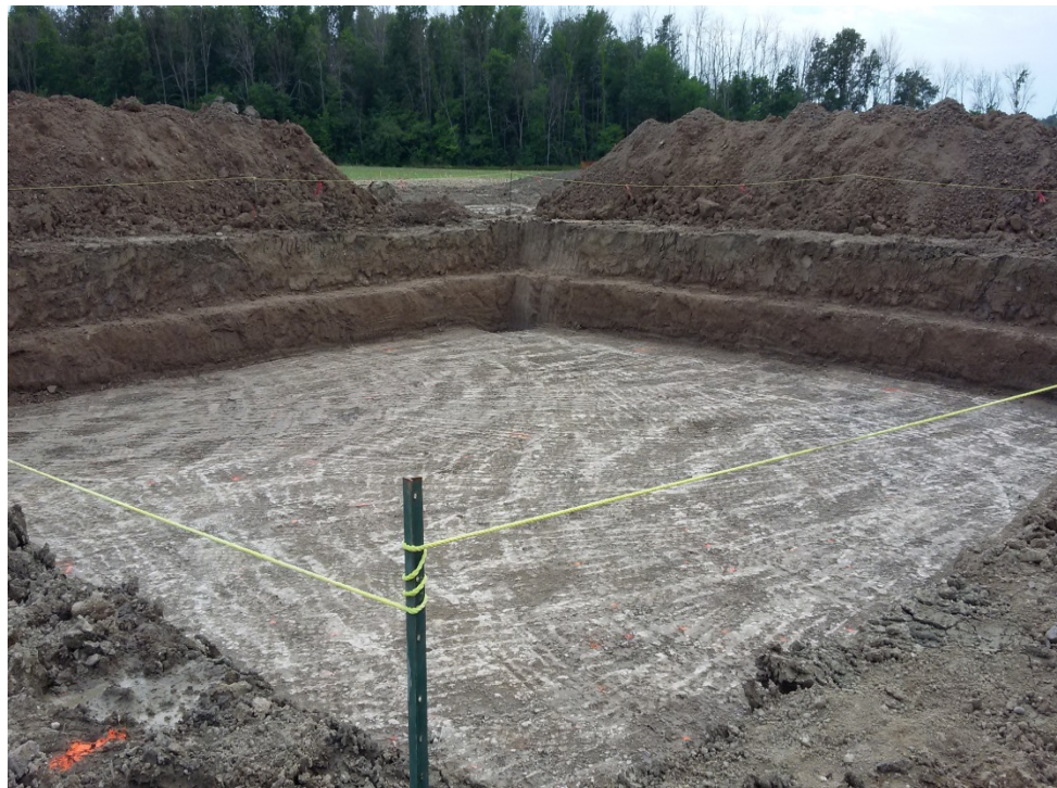
Photo 2 – CP233 – Foundation Subgrade
