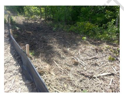
Photo 2: Typical Mulch Distribution and Silt Fence
