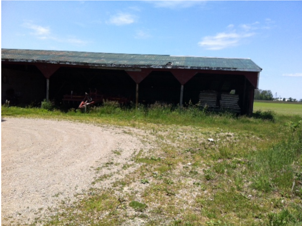
Plate 13: Area of previous disturbance, not assessed, facing west
