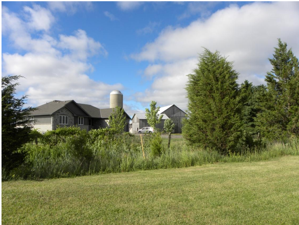
Plate 20: 3979 Michigan Line, 19 th century barn buildings situated alongside modern residential structure.
