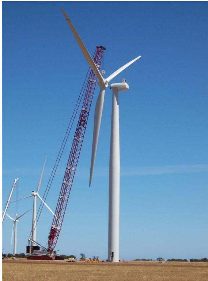
Figure 4.4-4: Example of a Crawler Crane
