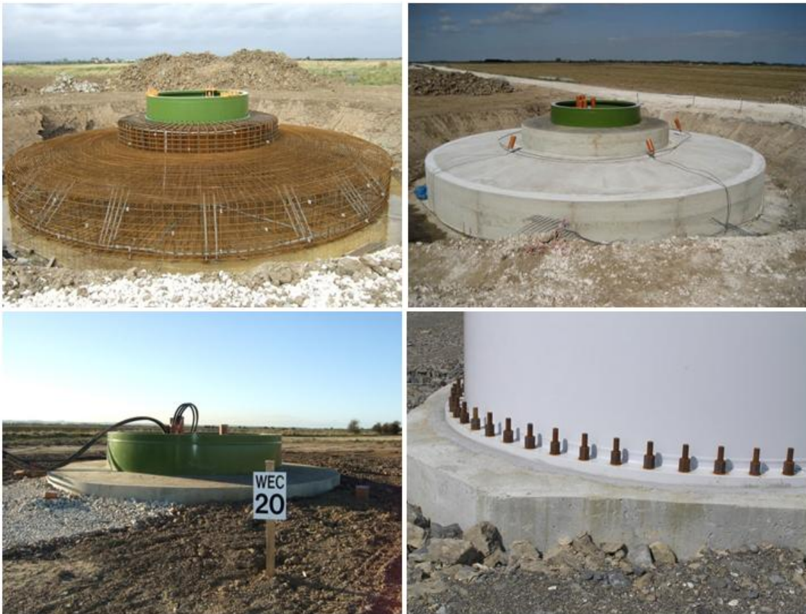
Figure 4.5-3: Example of Turbine Foundation Construction Stages
