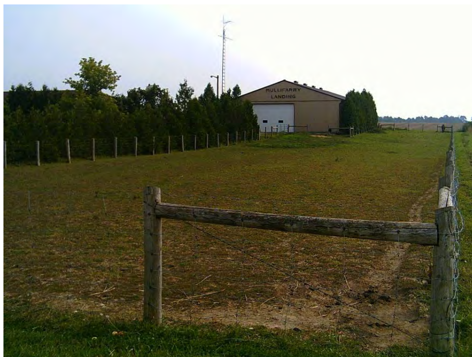
Figure 19: Barn Labelled “Mullifarry Landing” at 3003 Mullifarry Drive; Facing South from Mulifarry Drive
