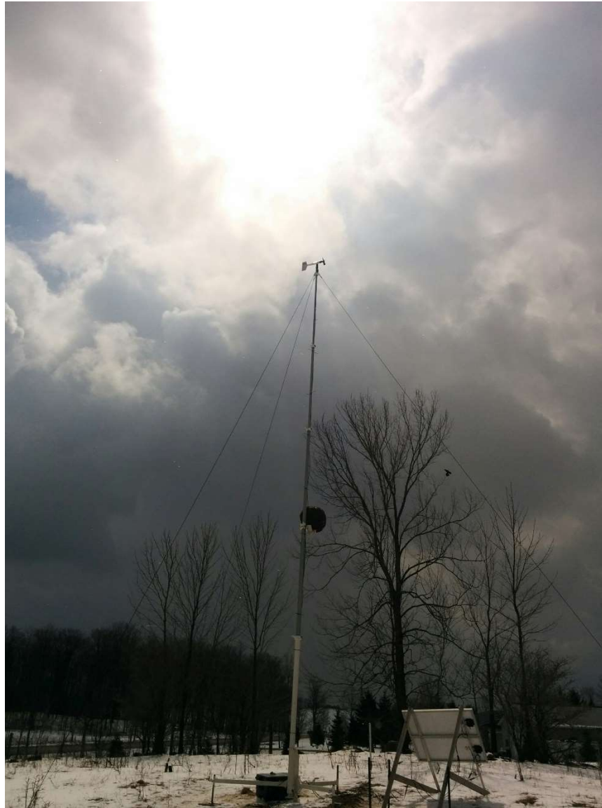
At 90° to the Line Between the Turbine and Measurement Location, Including Area in the Vicinity of the Microphone and the Receptor
