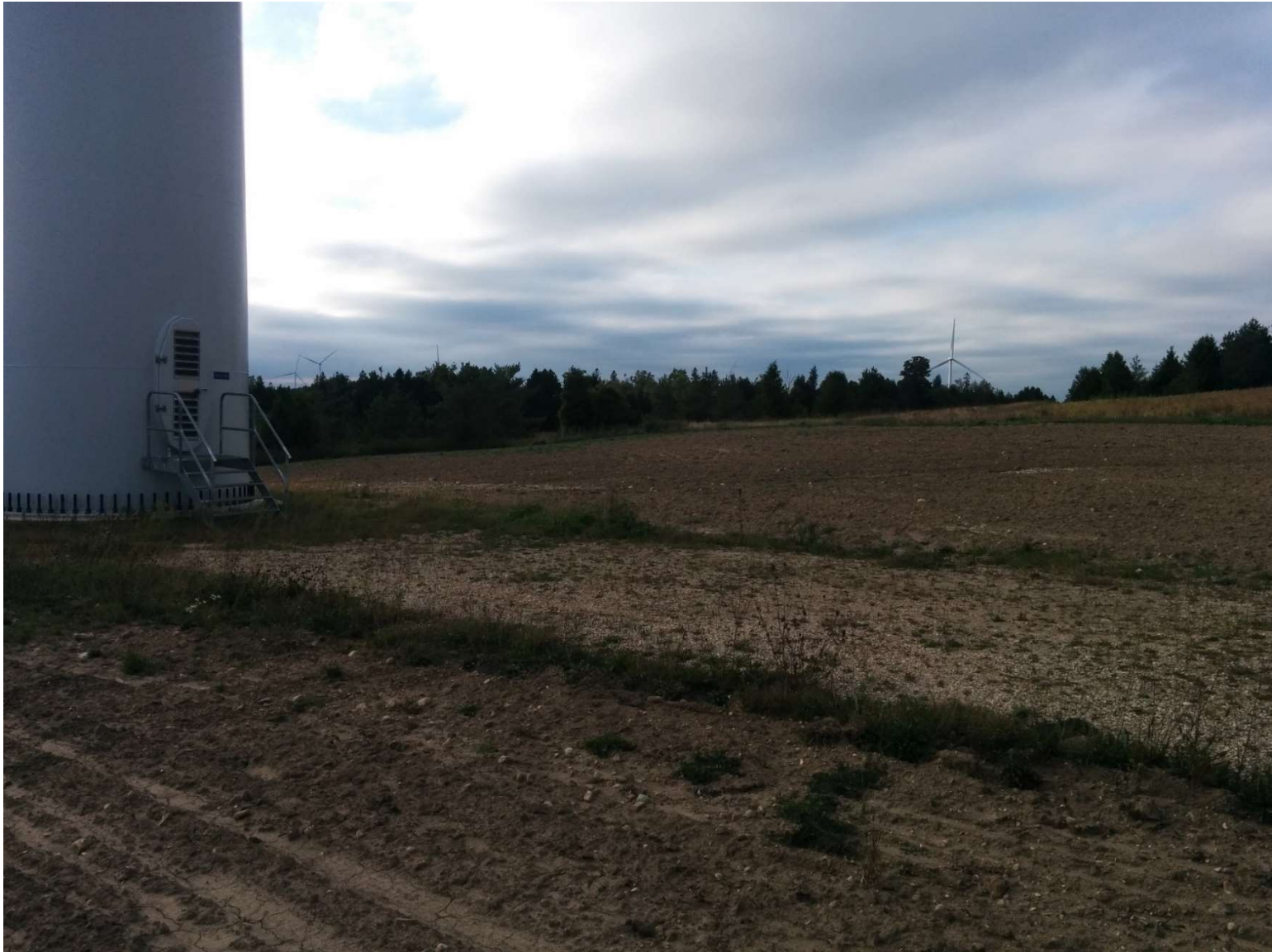
In Close Proximity to the Turbine in the Direction of the Measurement Location
